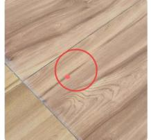
8 Crack / damage / bend observed in floor tile
